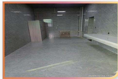
Renovation of staff shower facility 員工浴室整改
