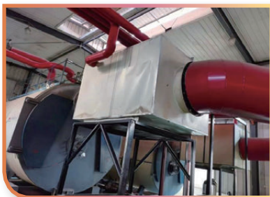
Gas boiler flue gas waste heat reused to heat boiler feed water, resulting in an increase of efficiency by approximately 3-7% 燃氣鍋爐煙氣餘熱再利用加熱鍋爐給水，效率提升約 3-7%
